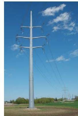
Figure 2: Steel Transmission Line Support Structure
