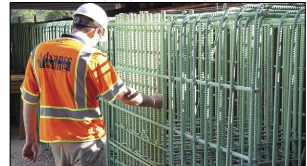
Rebar inspection at the replacement of twin bridges on Interstate 84..
