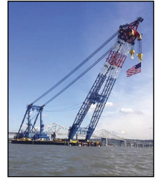
! Lift NY crane on $3.6 billion Tappan Zee Bridge replacement project..
